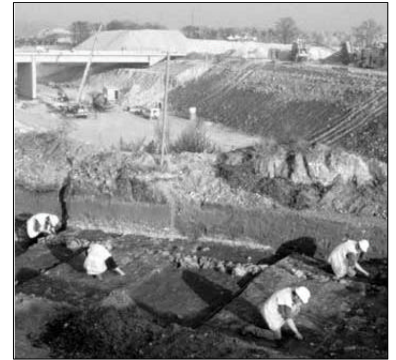
The excavation of the Roman Road at Roman Ridge. (Photo: P. Gwilliam)
